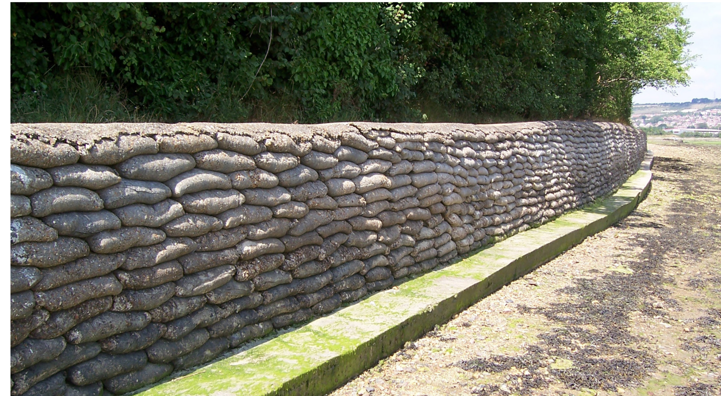
Concrete Bagwork Wall
