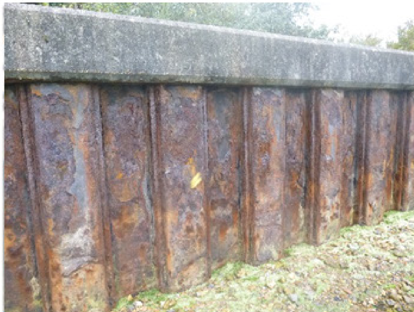
Steel Sheet Piling
