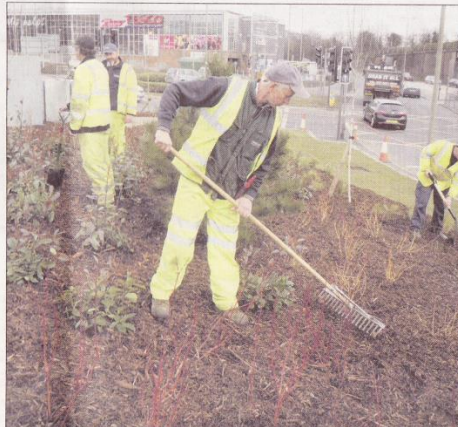
SMARTENED UP Men working on Quay Street Roundabout in Fareham
