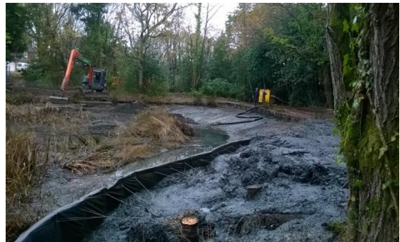
Coldeast: silt extraction & re-profiling
