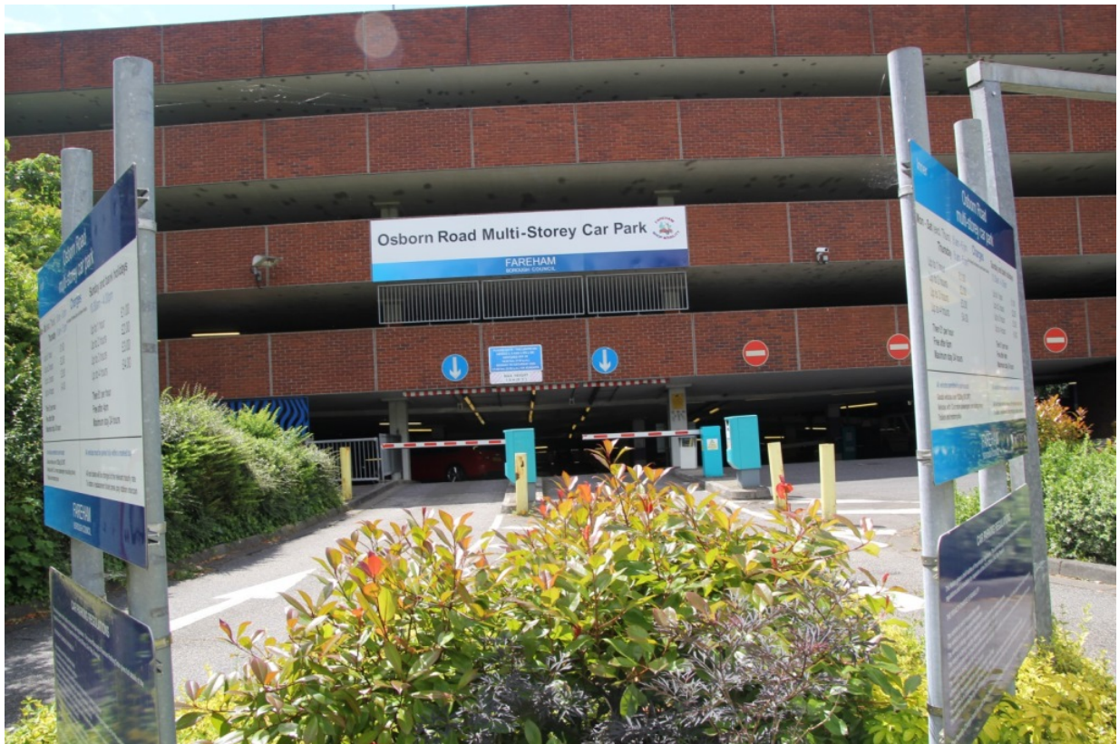
Osborn Road Multi-Story Car Park
