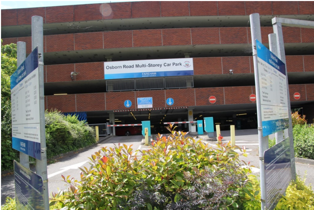
Osborn Road Multi-Story Car Park
