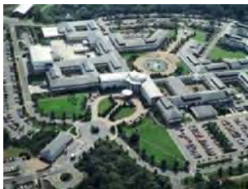
Cody Business Park, Farnborough
