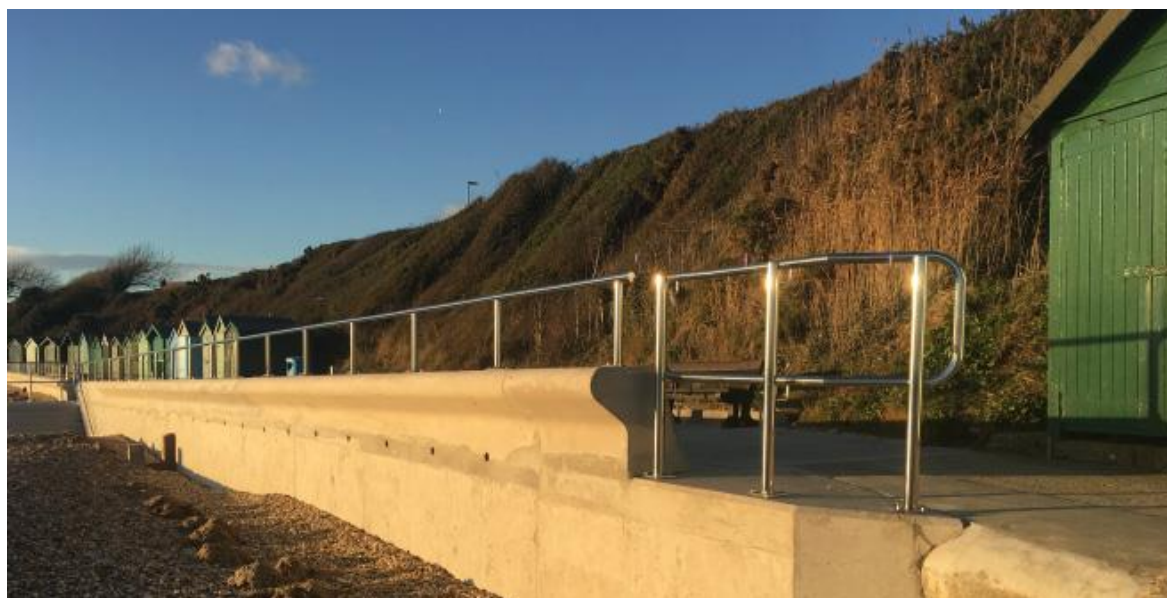
Completed Sea Defences at Hill Head
