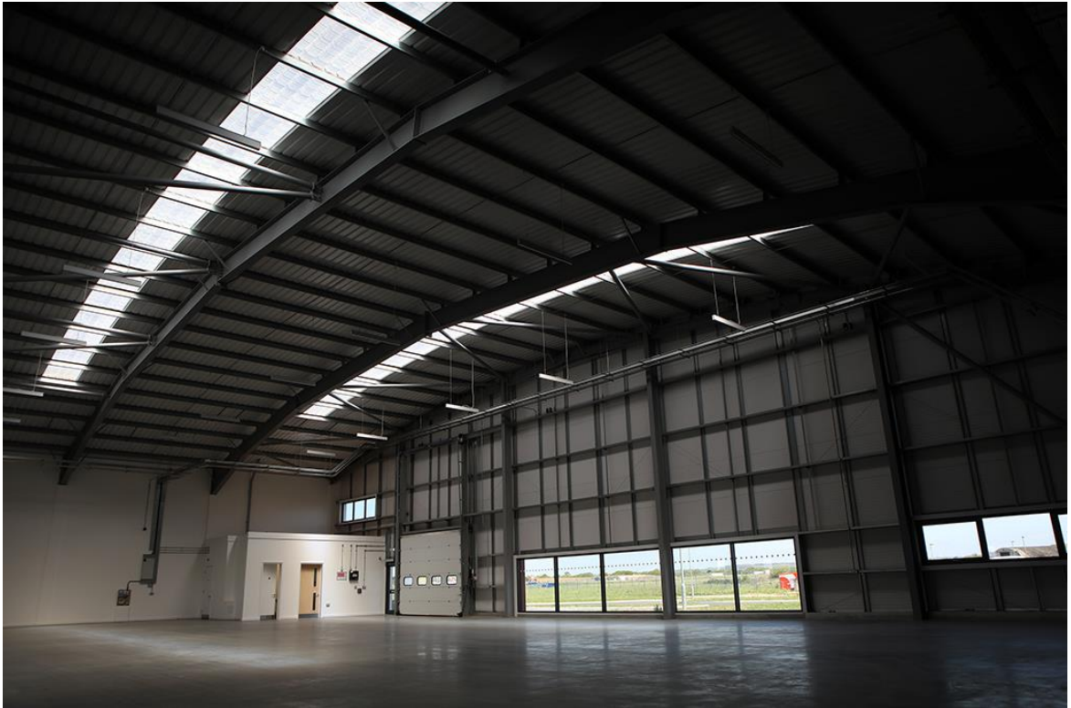
Hangar at Daedalus
