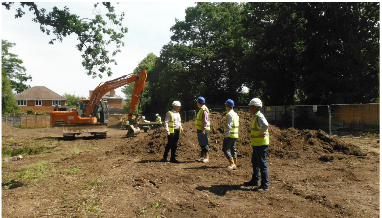
Land at Bridge Road - Fareham Borough Council affordable housing scheme now under construction
