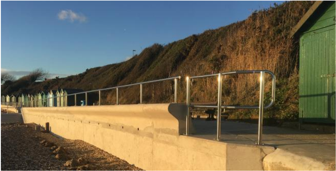
Completed Sea Defences at Hill Head
