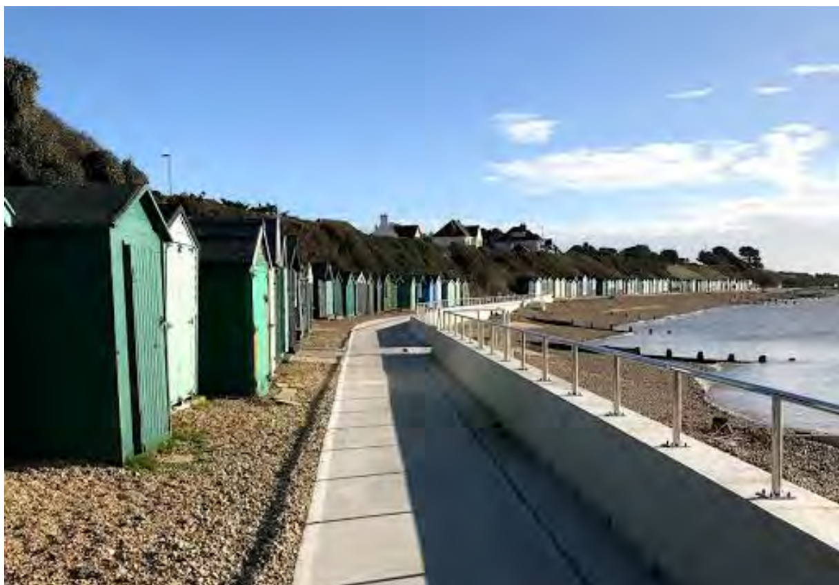
Hill Head sea wall replacement and promenade improvements
