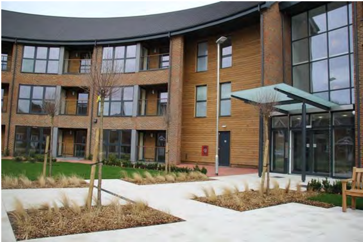
Sylvan Court, Fareham Borough Council affordable housing scheme – completed in this monitoring period.
