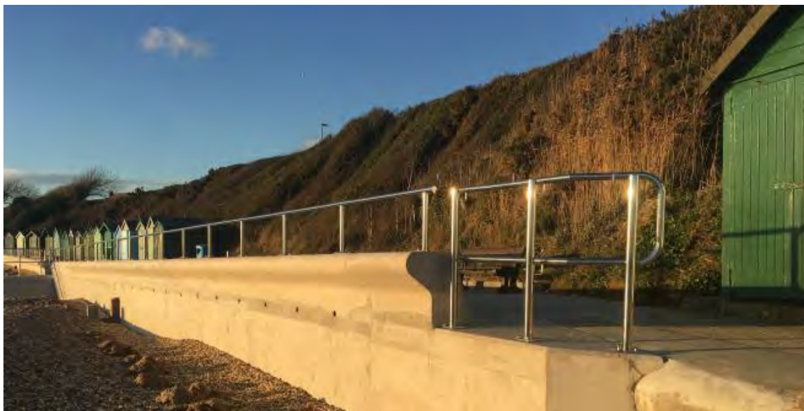
Completed Sea Defences at Hill Head
