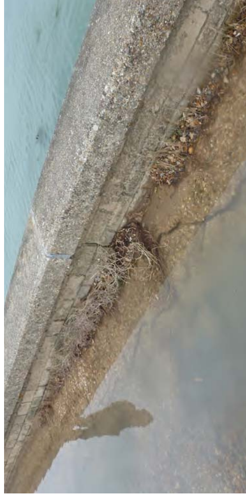
Sea wall at Hook Lake damaged by the winter 2013/2014 storms
