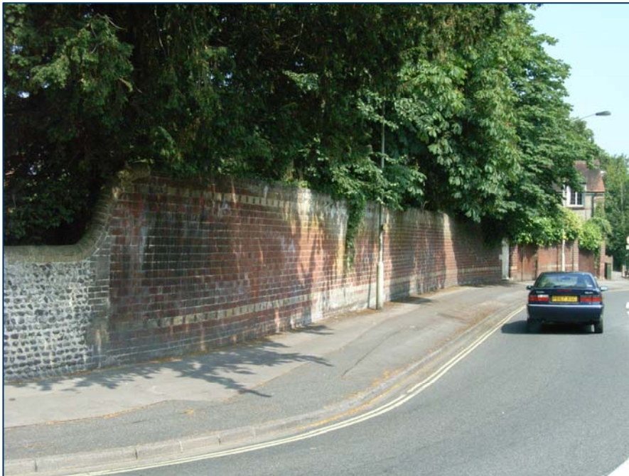
Figure 12: Rat trap bond wall with distinctive decorative string courses forming a very striking and attractive part of the local historic street scene in Fareham
