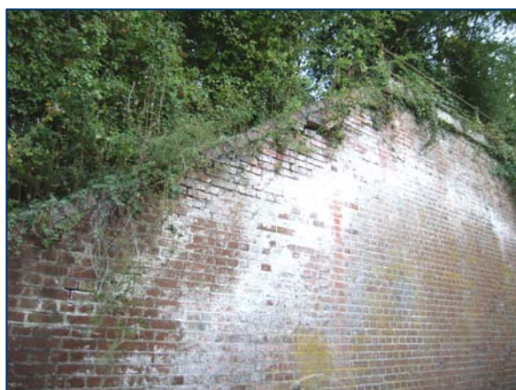
Figure 2: excessive vegetation to wall cappings
