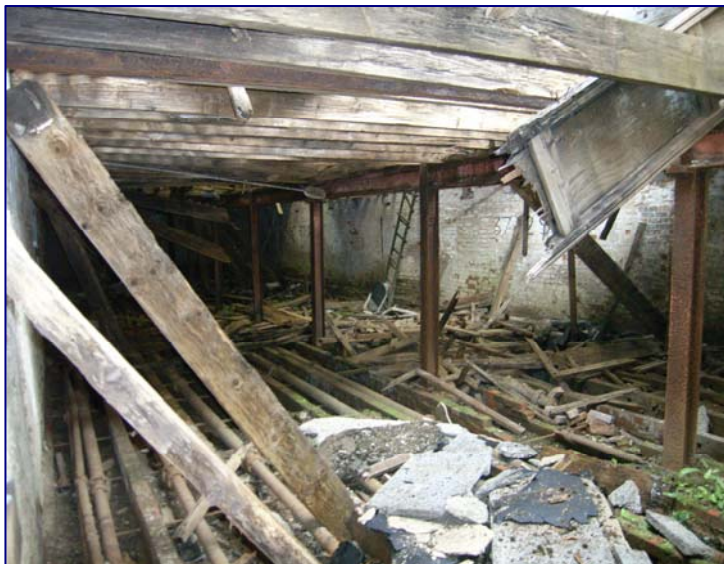
Figure 4: Drying shed 2 Burseldon Brickworks – roof has completely failed
