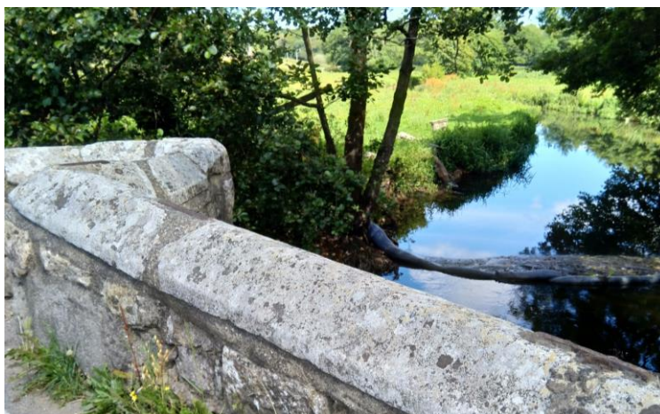
Figure 3.20 View upstream from Stony Bridge. Photograph: Deb McManus, July 2020.
