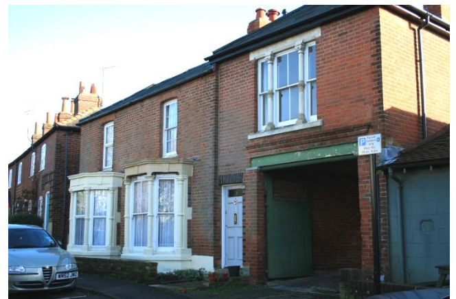
45 North Wallington –Formerly the Brewery Manager's House
