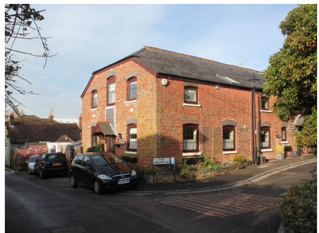
The former brewery, Drift Road
