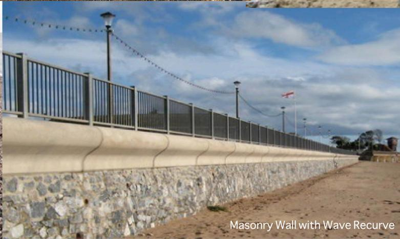
Masonry Wall with Wave Recurve
