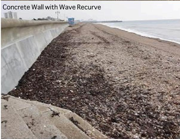
Concrete Wall with Wave Recurve
