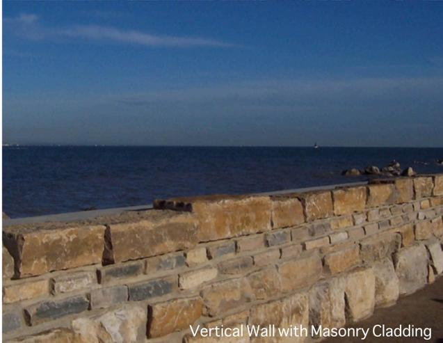
Vertical Wall with Masonry Cladding
