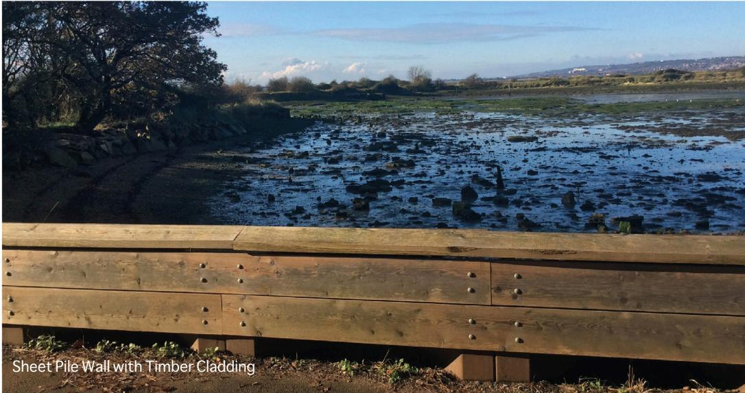
Sheet Pile Wall with Timber Cladding
