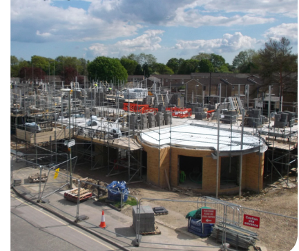
Collingwood Court in progress
