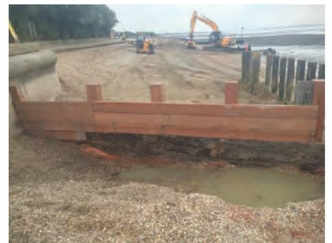
Phase 1 of the Hill Head project is now complete. New shingle has been laid and groynes have been rebuilt to help protect the promenade from wave damage.
