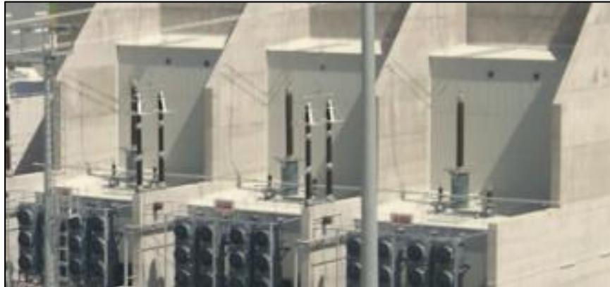
Figure 3 - Example of power transformer contained by audible noise enclosure
