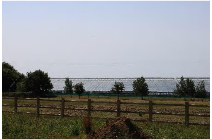
Figure 4.15 Photograph from Stubbington By-pass Construction site, looking South towards Glass houses on edge of Stubbington Photograph Charlotte Webb June 2020.
