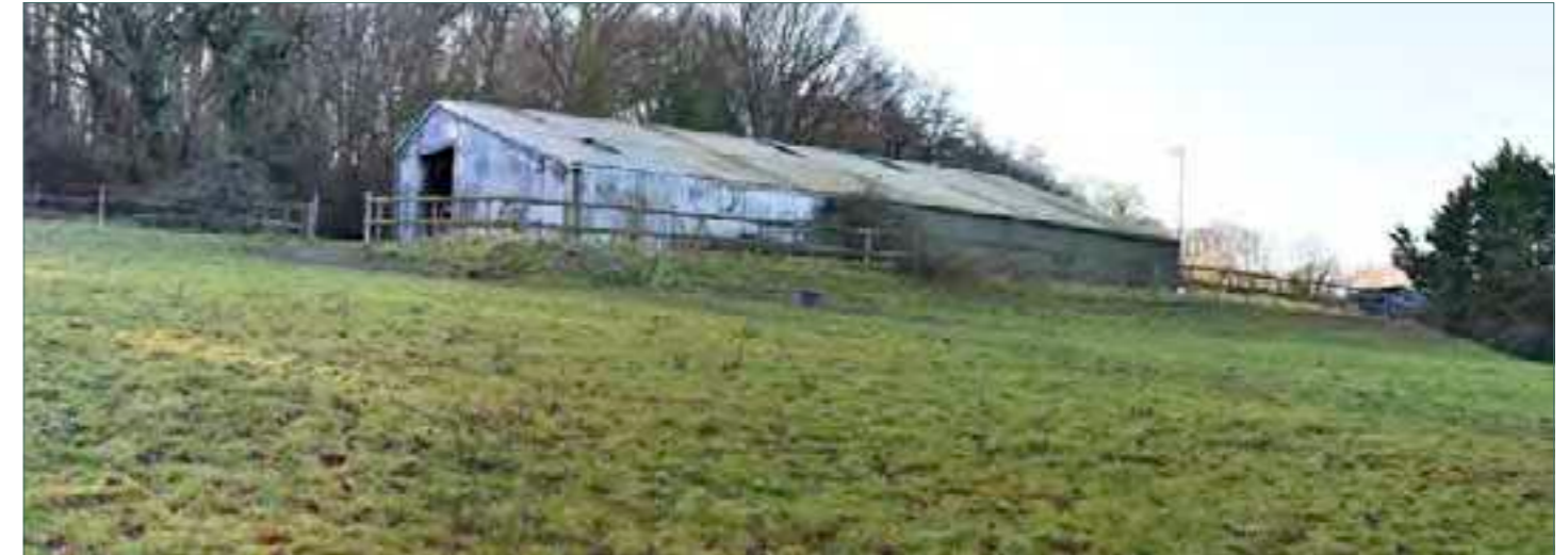
Photograph – Viewpoint S2 Winter View There is little change to the visibility across the Site in winter.
