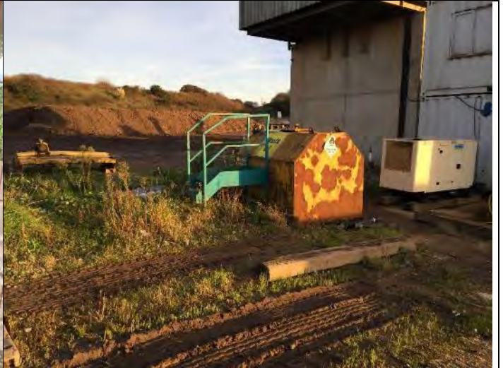
Photo 8: Waste oil storage tank at washing plant.
