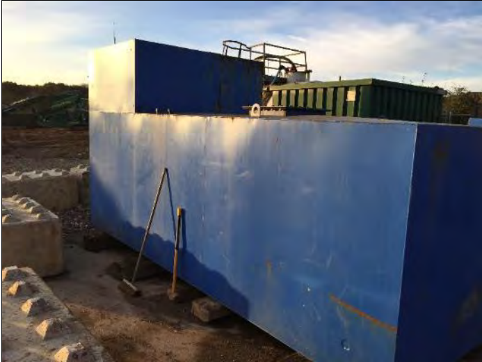
Photo 9: Above ground diesel tank at washing plant.
