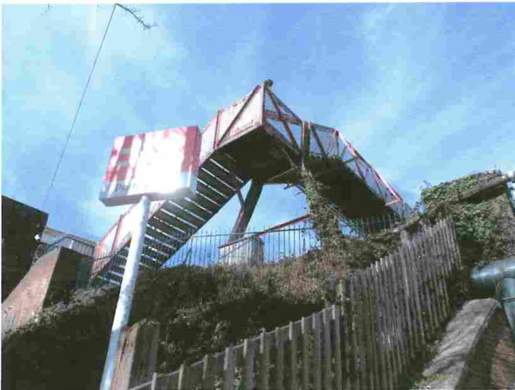
THE BRIDGE THAT HAS TO BE CROSSED TO NORTHERN SIDE PLATFORM
