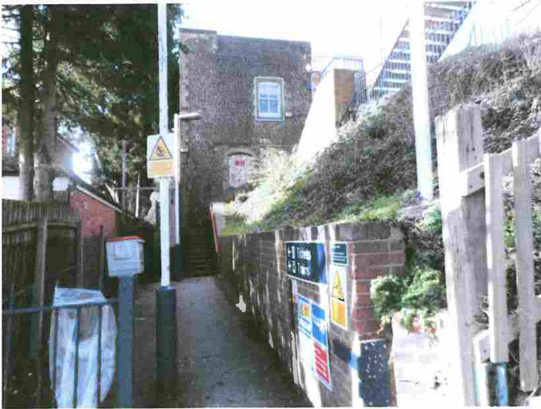
ENTRANCE ON THE SOUTH SIDE PLATFORM, 2 FLIGHTS OF STEPS TO THE TICKET OFFICE
