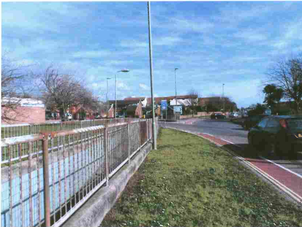
PHOTO 1. NO PAVEMENT ONLY A GRASS VERGE – LOOKING EAST.
