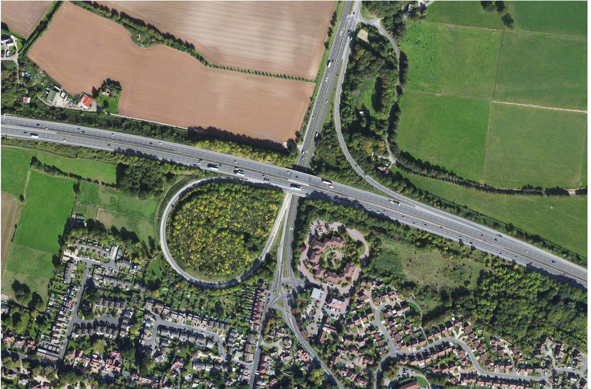
FIG 2.5 AERIAL VIEW OF M27 JUNCTION 10
