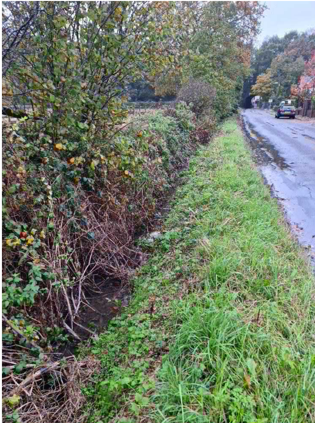
Photograph 1: Maintained ditch on Funtley Road.
