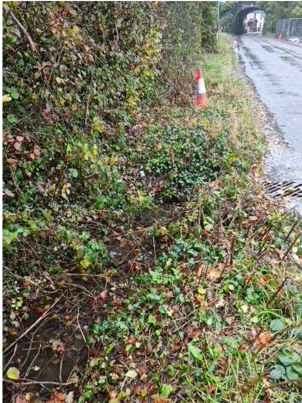
Photograph 2: Submerged 300mm diameter culvert and headwall.
