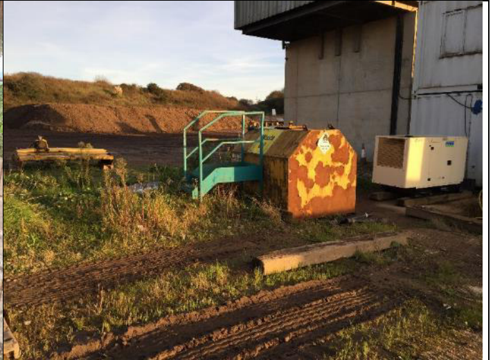
Photo 8: Waste oil storage tank at washing plant.
